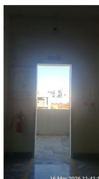
Emergency Exit 1.jpg
